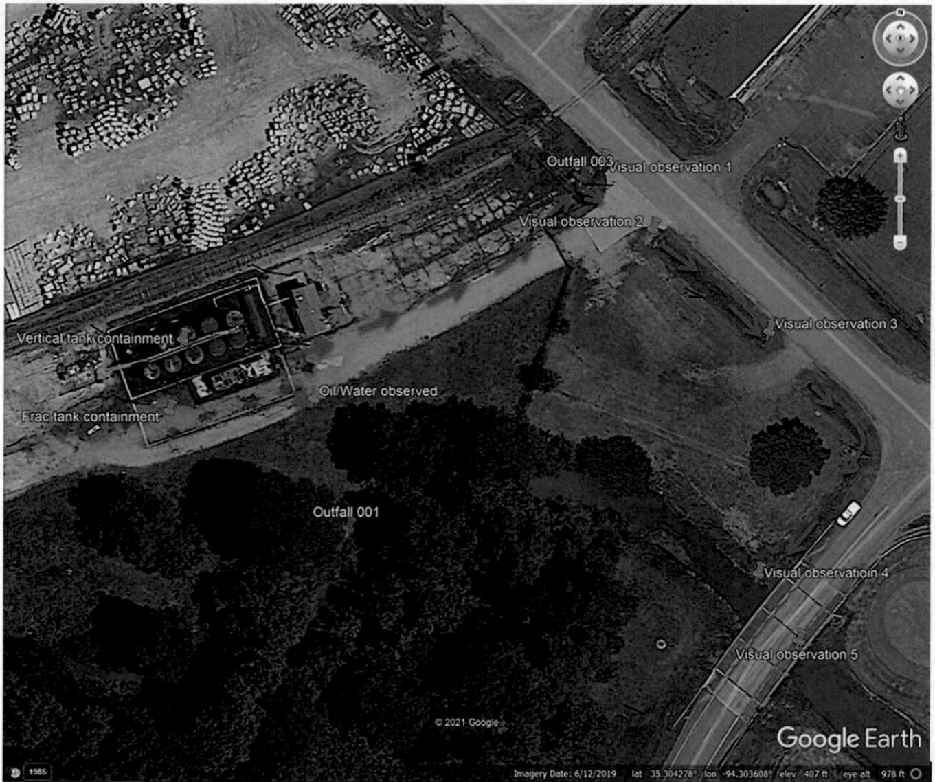
Figure 1. Google Earth image dated June 2019 showing the facility, flow path, and locations of visual observations.
